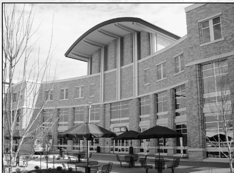
The $29 million Student Union (left) and complete renovation of the existing Reng Center (left) houses a new dining hall, meeting facilities, bookstore, computer labs, a food court and other features. Indian Village Apartments (above) accommodates up to 100 families. Collegiate Park (at top) serves 336 students.
